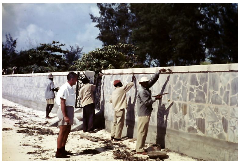
Zvonko inspects construction of the sea-wall protecting President's Jomo Kenyatta garden.
