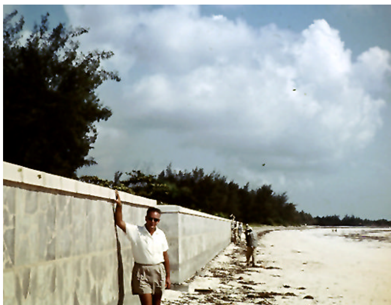
The sea-wall is almost completed as viewed northwards on the Bamburi Beach.
