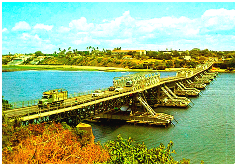
This pontoon bridge linked the mainland in background with the Mombasa Island. Whole traffic even the heavy lorries had to cross over this toll-bridge.
