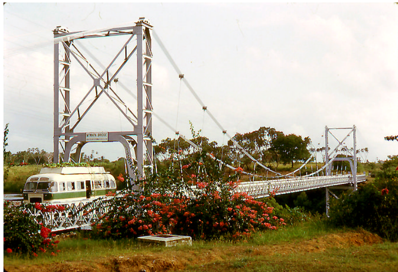
The toll-bridge over the Mtwapa Creek built from military parts known as the Bailey bridge.
